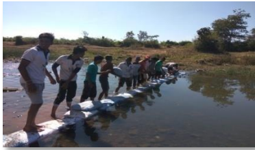
Construction of check dams
